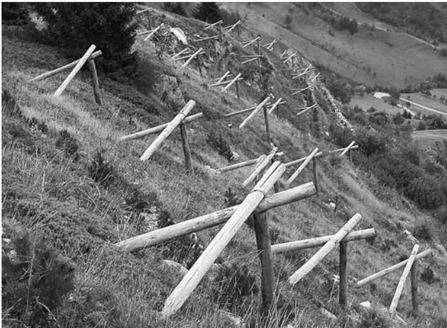
Fig. 3. Wooden tripods which prevent snow gliding and enable planted trees to pass the threatened juvenile phase. Vaujany, Savoie, France.
